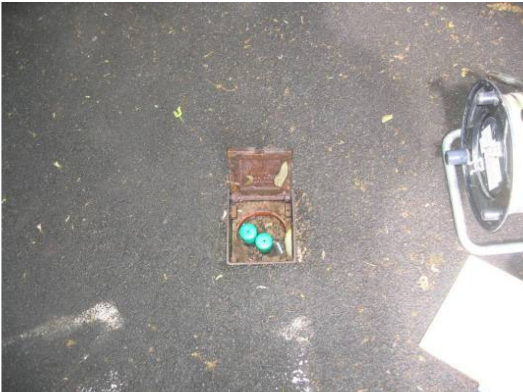
Plate 45 Scarborough South Cliff D2
