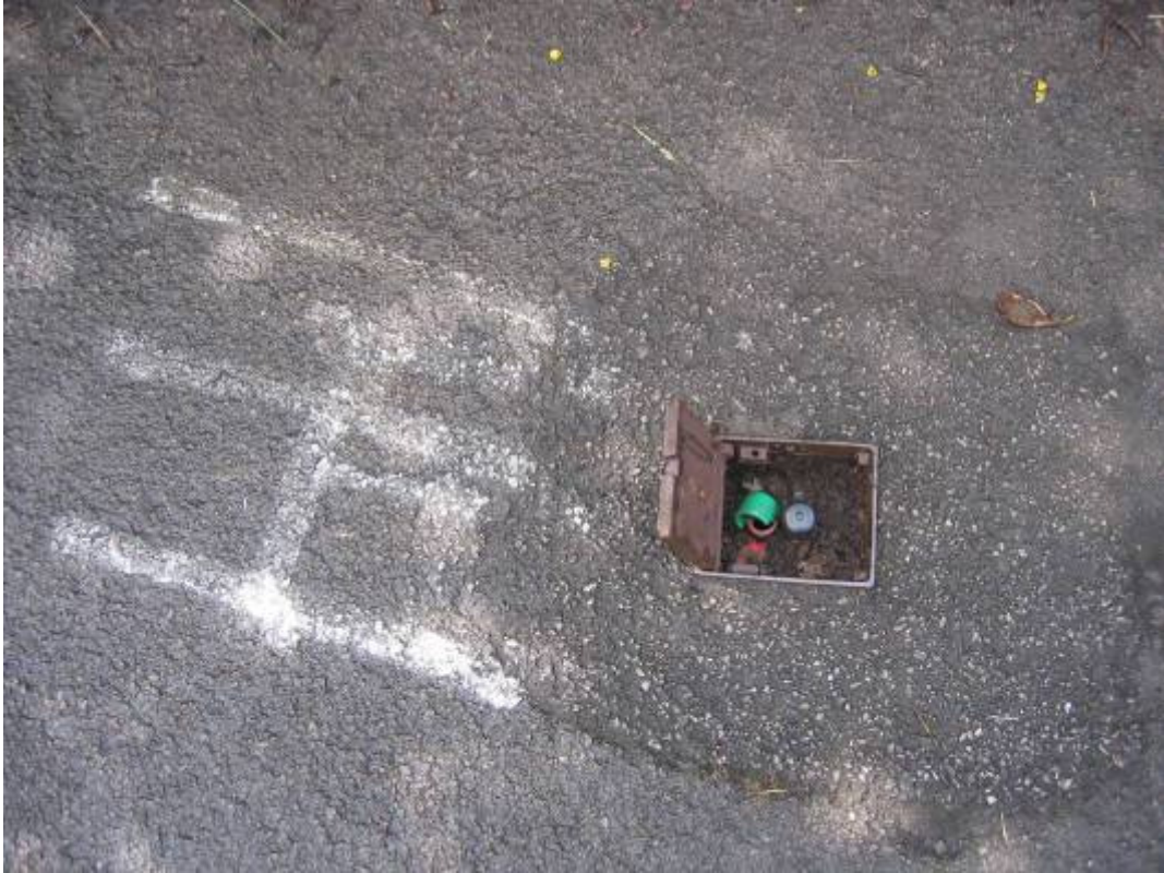
Plate 32 Scarborough South Cliff H1
