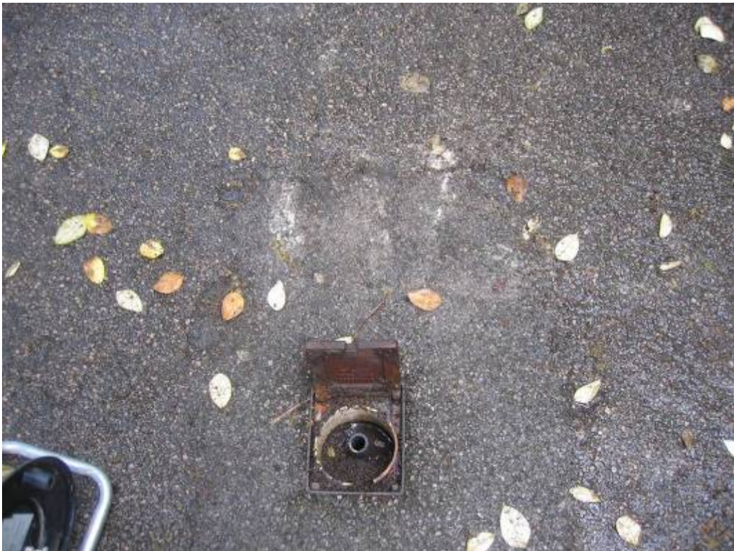
Plate 33 Scarborough South Cliff H5
